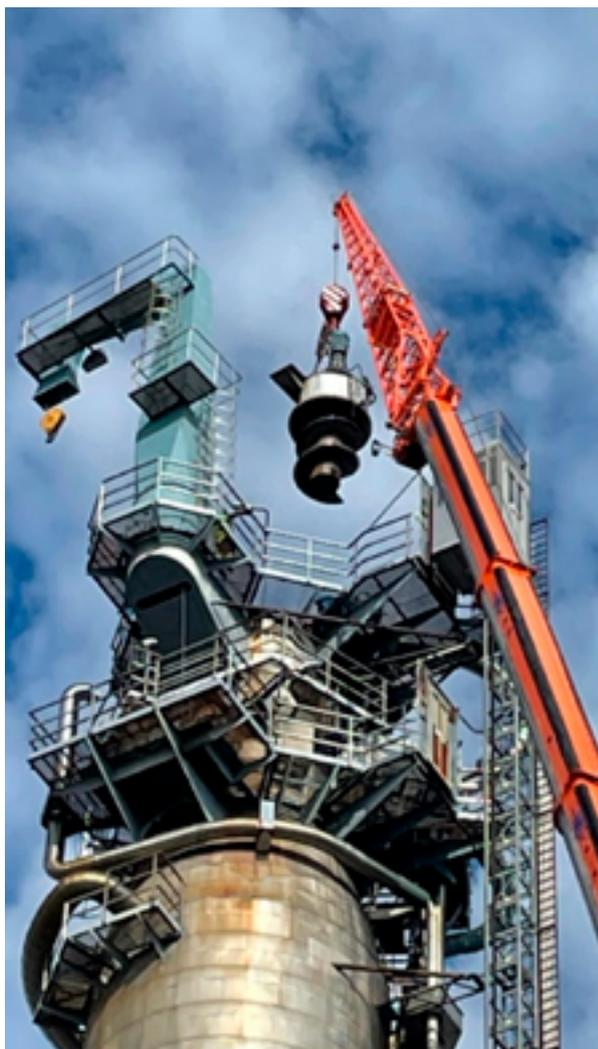
The old Luvo is lifted up through the roof of the boiler at Rottneros Mill.
